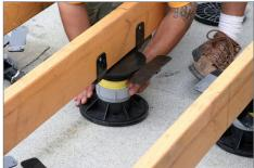
5. Bison Pedestals can be adjusted for height even after the Joist Tops.
