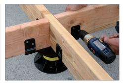
6. The Joist Tops can accomodate either 2x or 4x lumber at 90° angles in all four directions.
