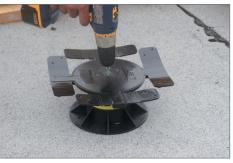
2. Screw Joist Top attachment into Pedestal using the Bison provided screw.
