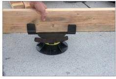
3. Place joist (2x or 4x) on top of the Bison Joist Top.
